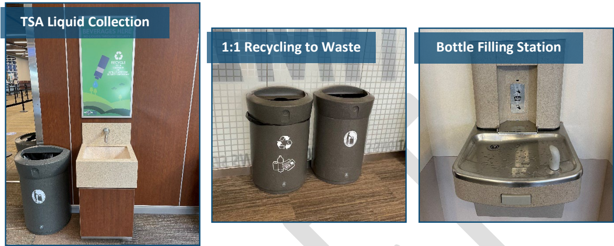
Figure D-8 Existing FSD Infrastructure – Best Practices Achieved by FSD
